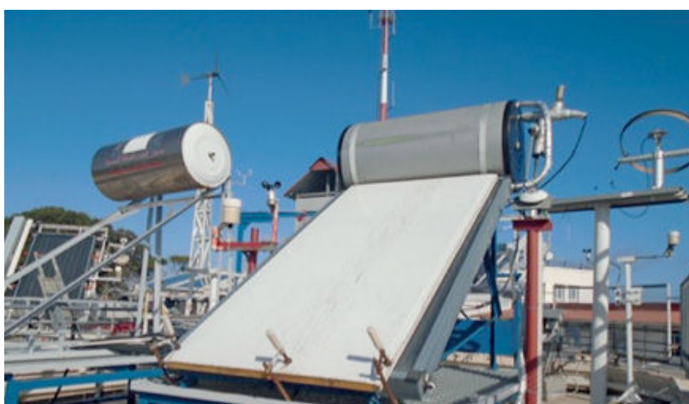
Figure 15: CDER - LEsS Lab in Algeria
