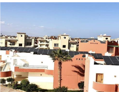
Sharm Bride 682 kWp
